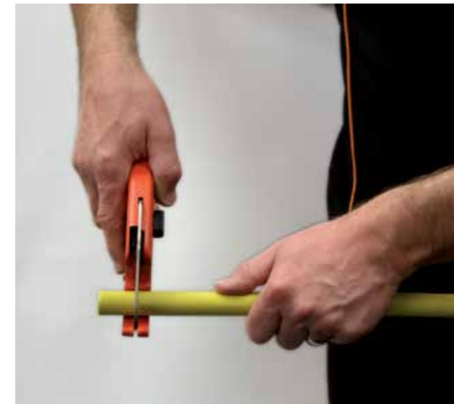
1. Cut pipe at right angle.
